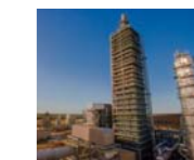
2016 Completed one of the world's largest flue gas CO 2 capture plants for enhanced oil recovery in the United States
