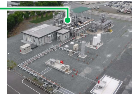
View of pilot plant (within JERA Shin-Nagoya Thermal Power Station)
