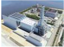
GTCC power generation facility
