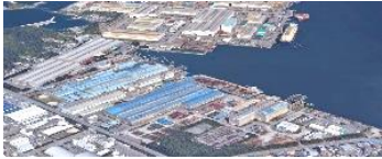
Koyagi Plant, Nagasaki Prefecture
