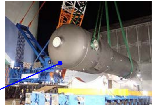
Steam Generator Replacement (SGR)
