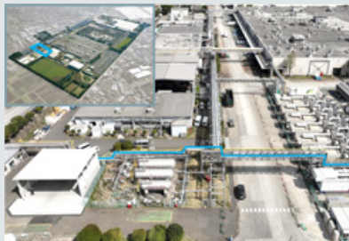
Hydrogen engine generator set demonstration facility
