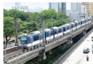
Manila Metro Rail Transit System Line 3 (MRT-3)
