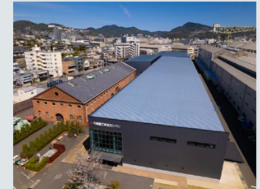
MHIAEL Nagasaki Plant
