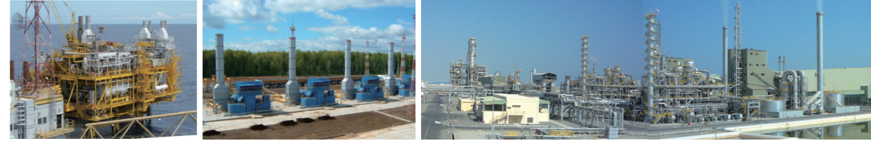
Offshore gas treatment plant
