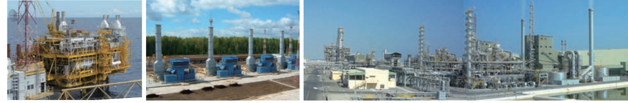
Offshore gas treatment plant
