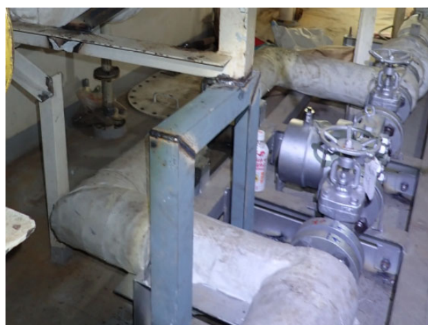
Steam Inlet Line and Drain Line Added with the Hot Standby Function
