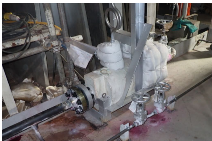
Steam Inlet Line and Drain Line Added with the Hot Standby Function
