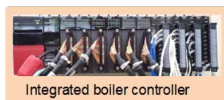
Current model PLC after replacement
