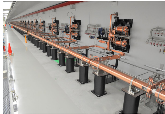
Figure 9: Installation of C-band section (by RIKEN).
