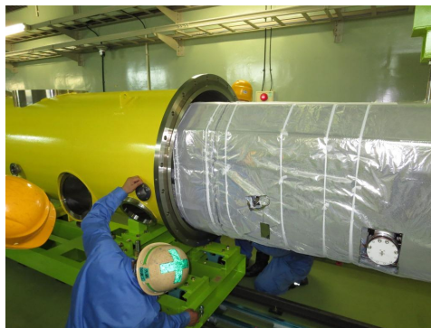
(a) Assembly of vacuum vessel
